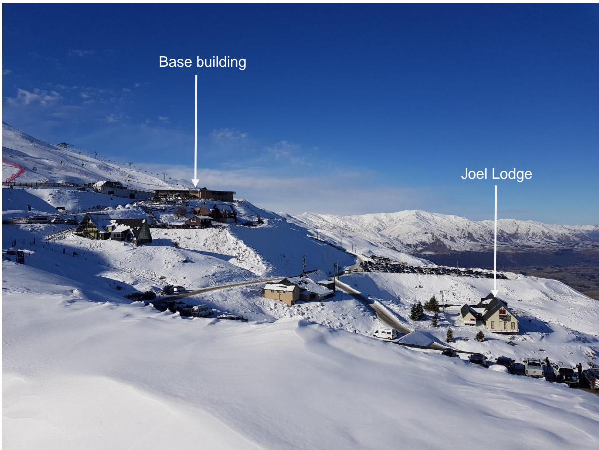
Winter view of Coronet Peak base area, with annotations showing the main base building and Joel Lodge. Photo credit: Gregor Macara.
